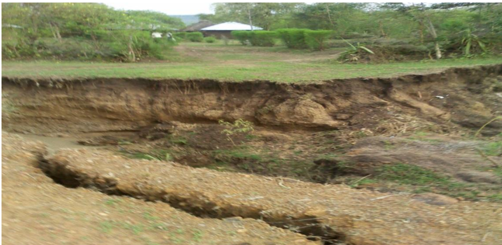
Picture 1: Homesteads facing imminent collapse.
